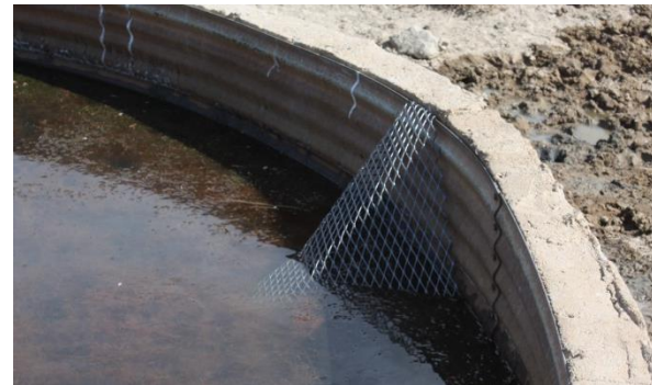
Properly installed stock tank ladder (photo courtesy of the Colorado Prairie Initiative)
