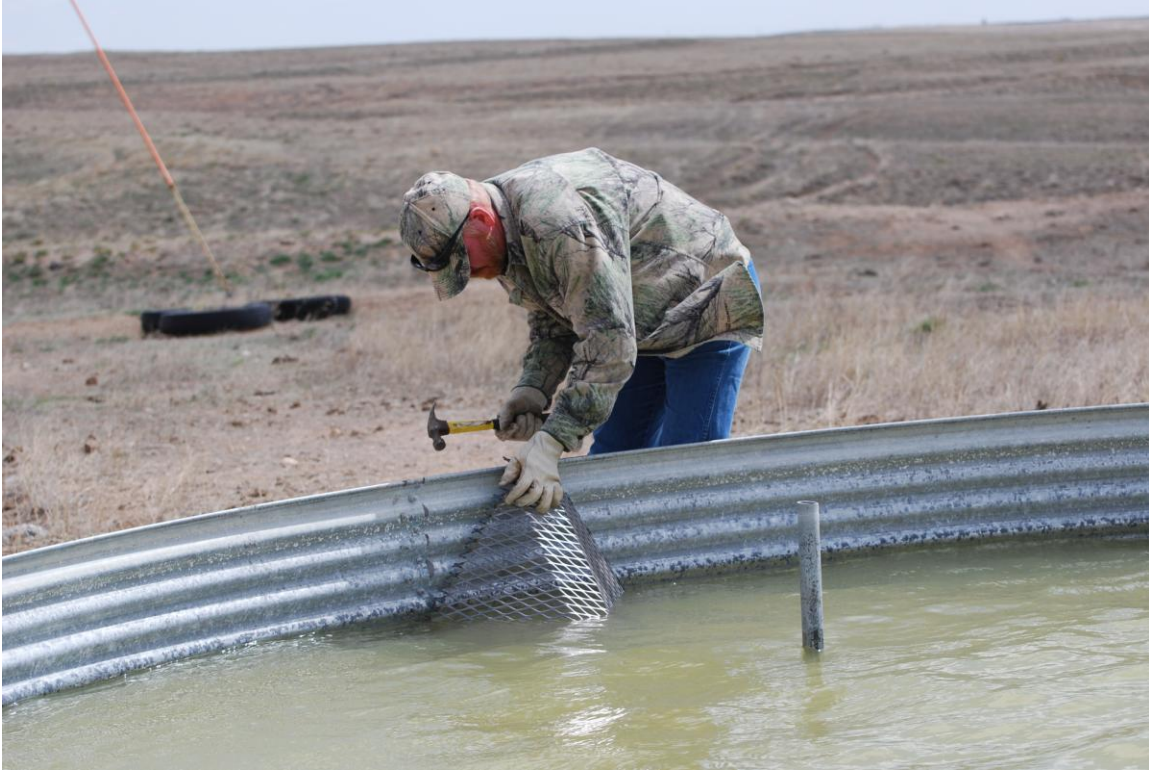
Figure 12. Nebraska Prairie Partner Project Assistant, Larry Snyder, installing a wildlife escape ladder in a stock tank on a habitat project near Kimball, Nebraska, in April 2008.
