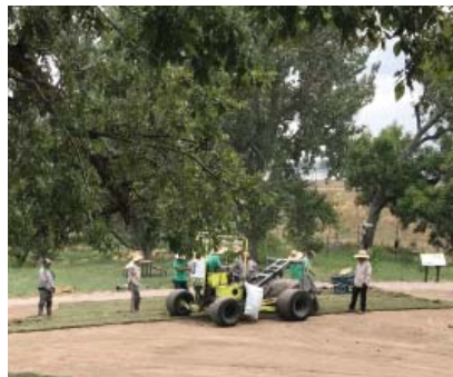
Installing buffalo grass sod on the freshly-scraped earth
